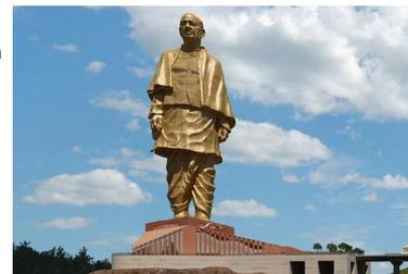
It took around 210,000 cu.m. of cement concrete, 18,500 tonnes of reinforced steel, 6,500 tonnes of structural steel and 1,700 tonnes of bronze to build the statue. The statue has been engineered to withstand wind speeds of up to 50 m per second (almost 180 km/hr. ). The Statue can also survive earthquakes measuring up to 6.5 on the Richter Scale, at a depth of 10 km and within a radius of 12 km.
